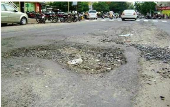
Fig. 1: Condition of roads with potholes.
